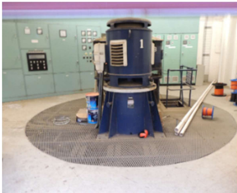
Figure 3 – Shaft A Bathurst Old Pump Station
