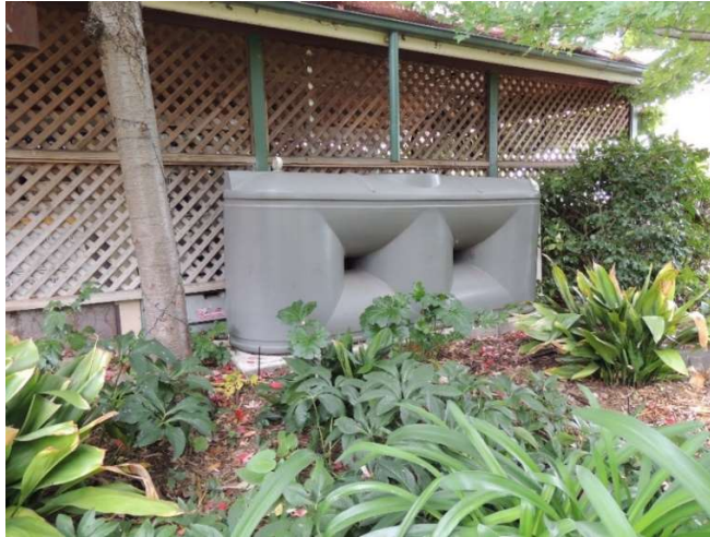
Figure 6 – 2000L rainwater tank
