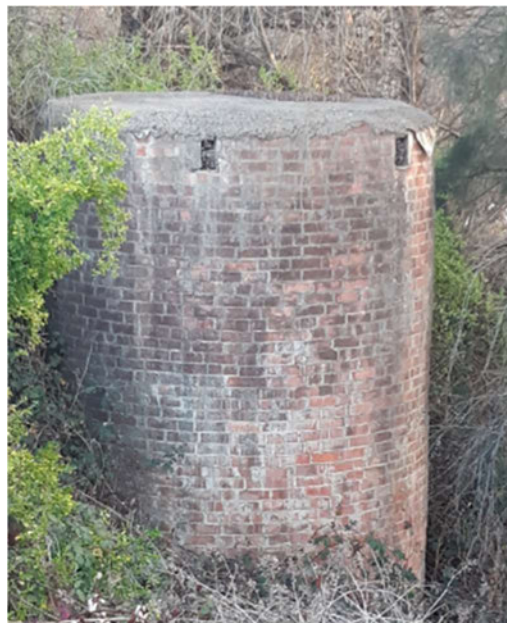
Figure 4 – Tunnel Air Shaft B
