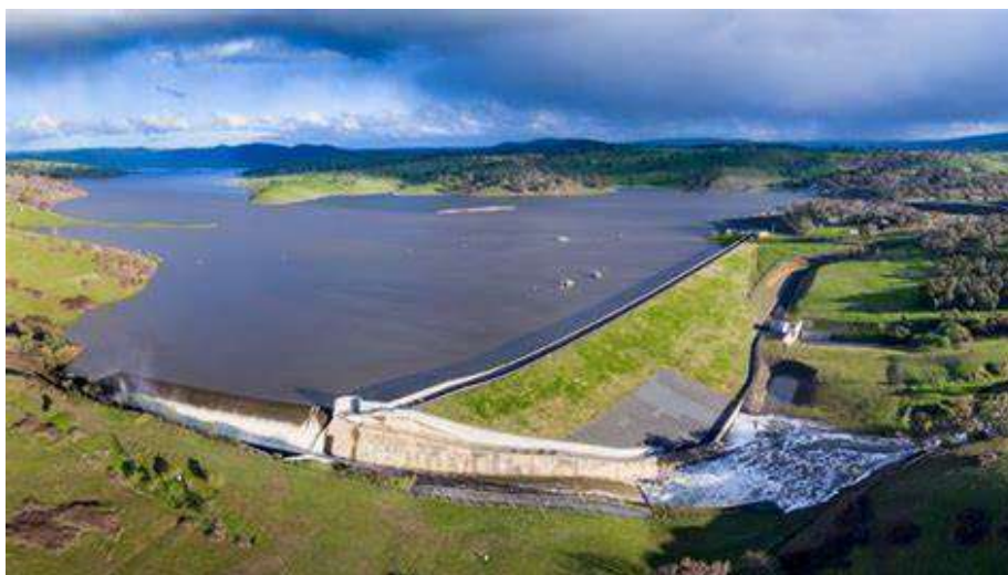
Figure 9 – Chifley Dam Showing Overflow Spilling
